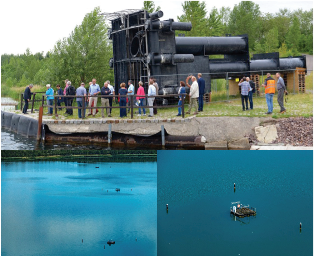
Figure 2 Deep water aeration system, top: on shore during renovation in 2017 (image: Christian Bedeschinski), bottom: in operation in 2019 (image: Peter Radke).
