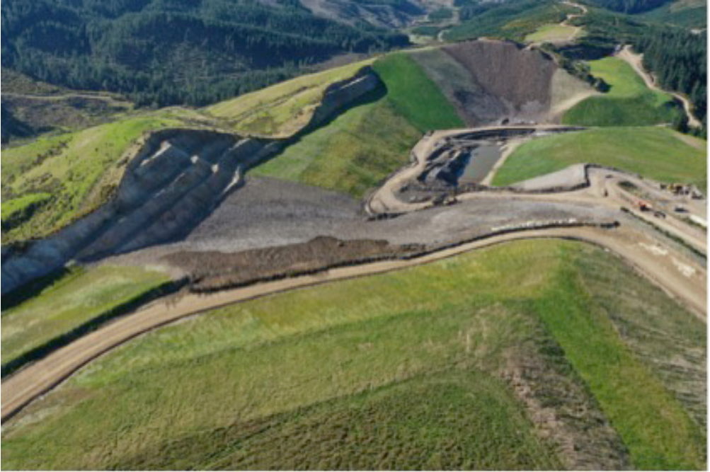
Figure 12 Site View showing final rehabilitation efforts and the N02 Pit Pond area.
