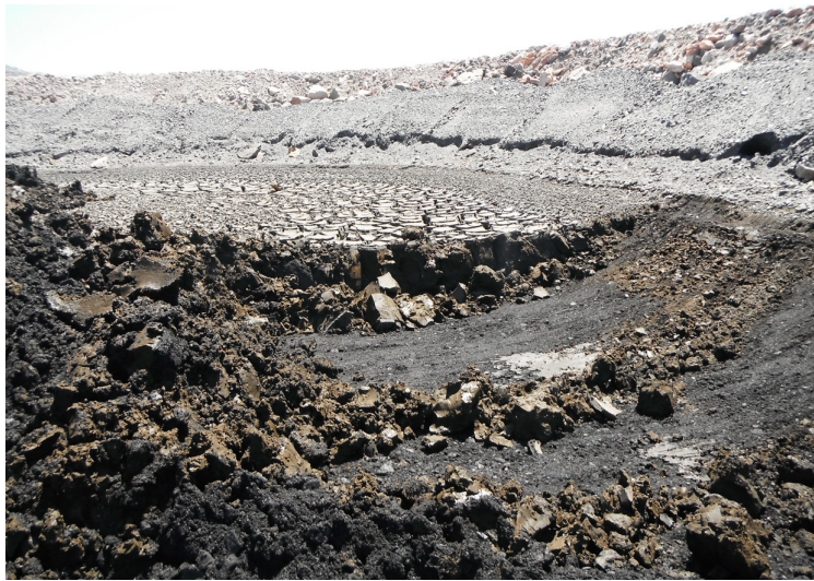
Figure 2 Dewatered sludge being removed from within a filter bed
