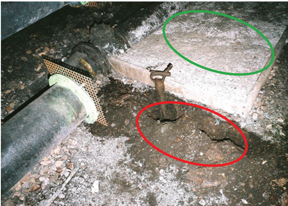
Figure 2 Example for the examination of the gallery floor around a former winder site.
