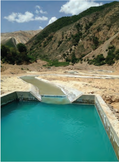
Figure 5 Open lime-zeolite channel system after construction
