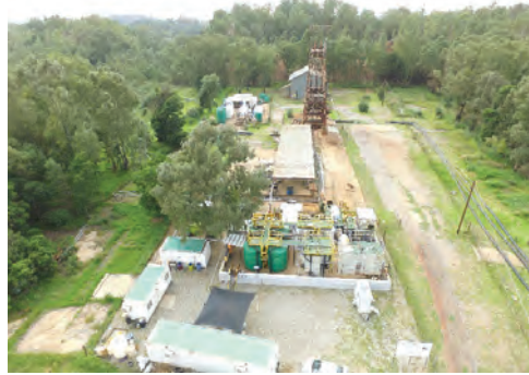
Figure 2 Aerial view of SAVMIN™ demonstration site
