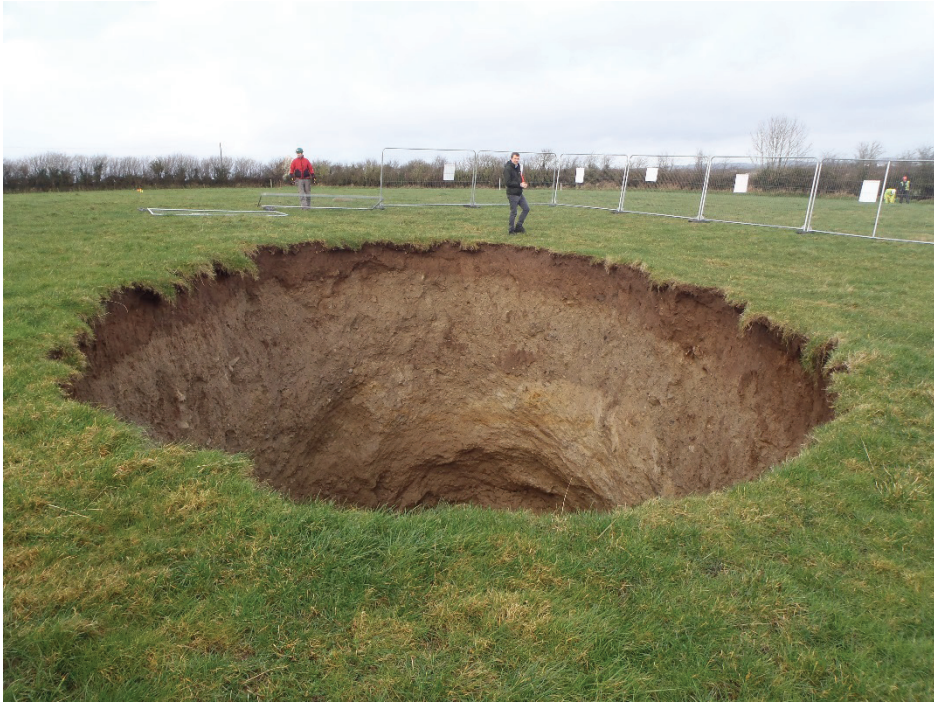
Figure 1 Sinkhole a few days after development.
