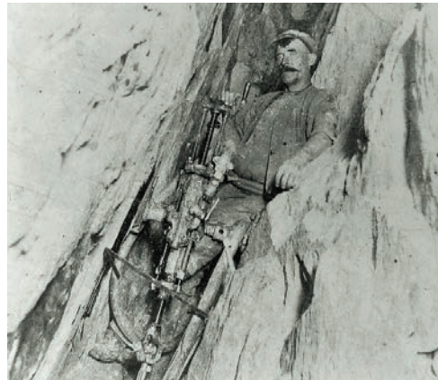
Figure 2 Steeply dipping slope in an early Witwatersrand underground mining operation (Ball 2015)
