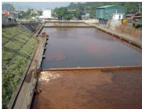
Figure 5 Equalizing reservoir in Nui Nhen MWTP, Quang Ninh
