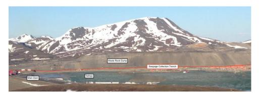
Figure 9 – Tailings facility and waste rock dump
