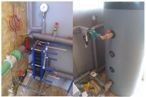
Figure 3 Pilot installation of heat pump in Armada Development (fot. M. Glodniok).
