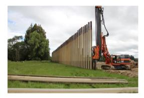
Figure 16: Sheet pile installation with RG 19T
