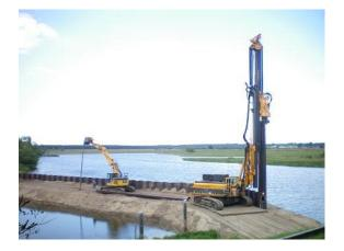
*Figure 15:* Construction of a ship lock near Quitzöbel, Germany. Sheet pile installation with RTG RG 19T and Top Vibrator MR 105 V
