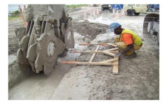
Figure 11: CSM installation with RG 25 S
