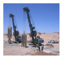
Figure 8: Cut-off wall installation BAUER GB 60
