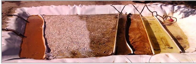
Figure 3 Mine water passive treatment pilot plant
