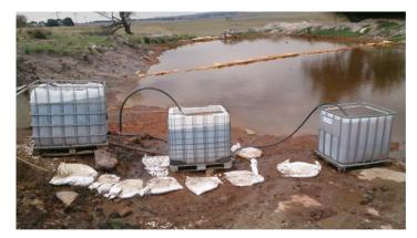
Figure 2 Carolina pilot passive treatment RAPS and oxidation units
