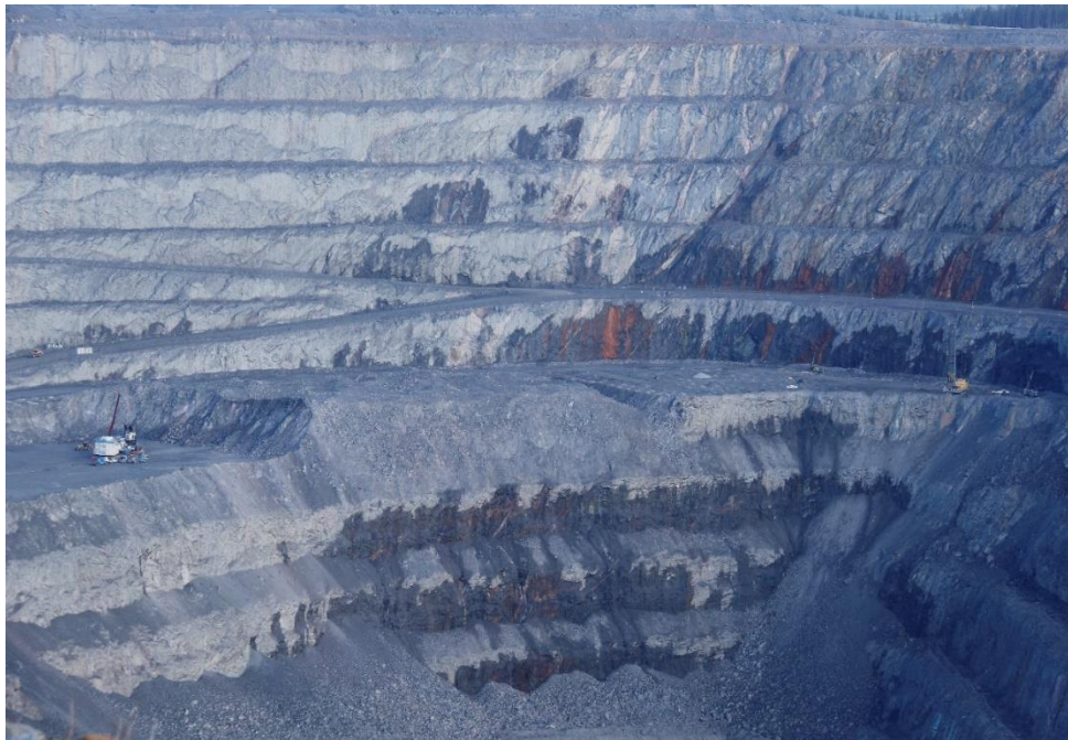
Figure 1 Wet and dry zones in Aitik north pit, Photo by Lars de wall
