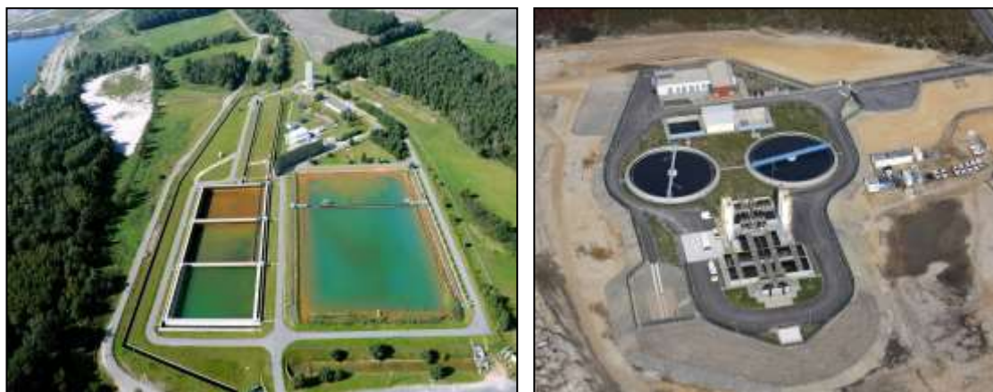
Figure 3&4 Central water treatment plants in Lusatia „Rainitza“ and „Am Wolkenberg“, pictures by Peter Radke LMBV and Vattenfall EM.
