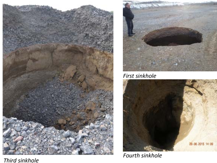
Figure 3 Views From the Sinkholes Developed in the Study Area
