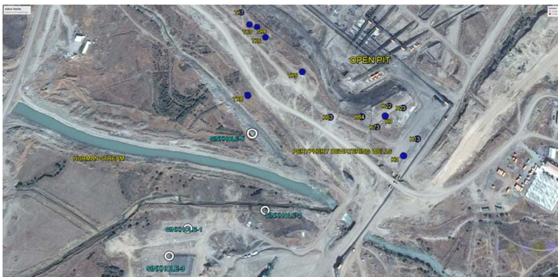
Figure 2 Location of the Sinkholes in Relation to the Open Pit.
