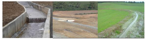
Figure 7 Aljustrel cleanwater diversion channel and Vale d'Abrutiga surface run-off drainage system.
