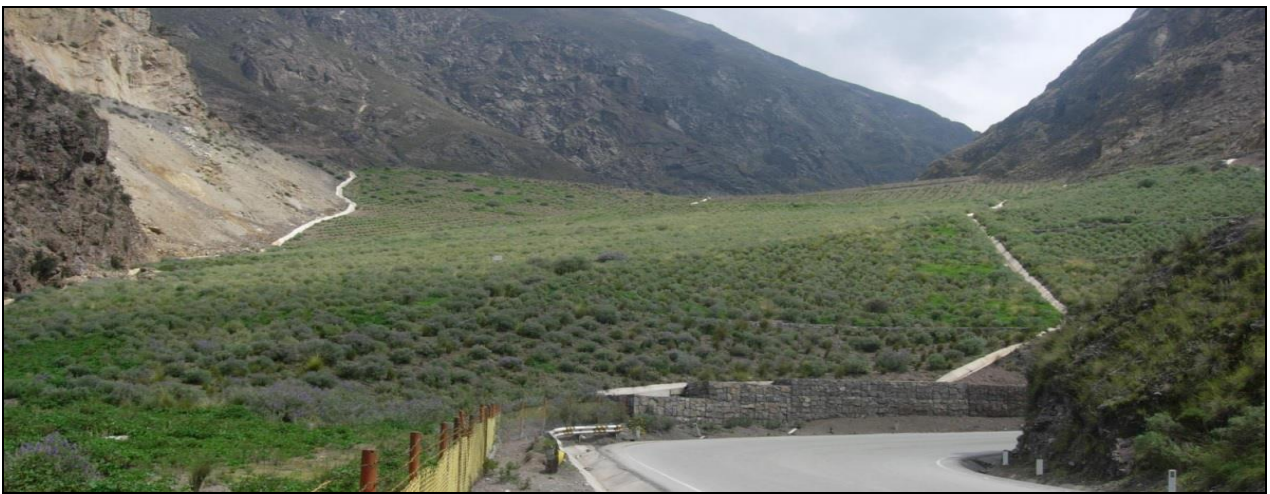
Figure 10 Tablachaca TSF closure overview (Estrella, 2008)
