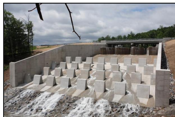
Figure 2 Spillway and Energy Dissipators
