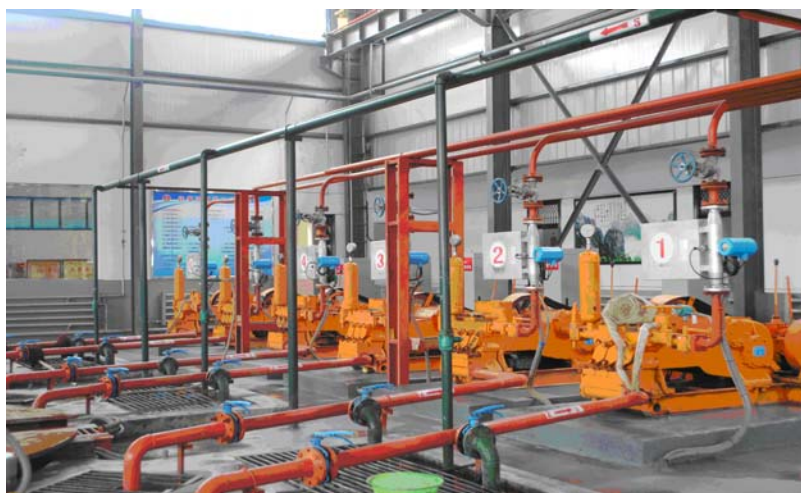
Fig.6 Ground grouting station
