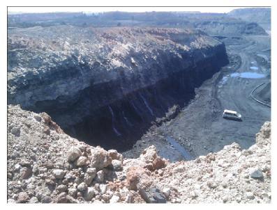
Fig. 4 Seepage from the high wall
