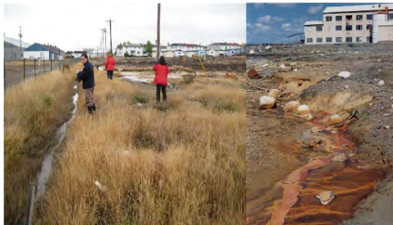
View of drainage ditch toward Buchans River constructed with a phosphate waste drainage barrier in 2009 on the left. View of same ditch toward mill building on the right – (opposite view compared to left) in 1994.
