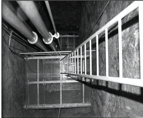
Figure 5. New shaft fixtures.
