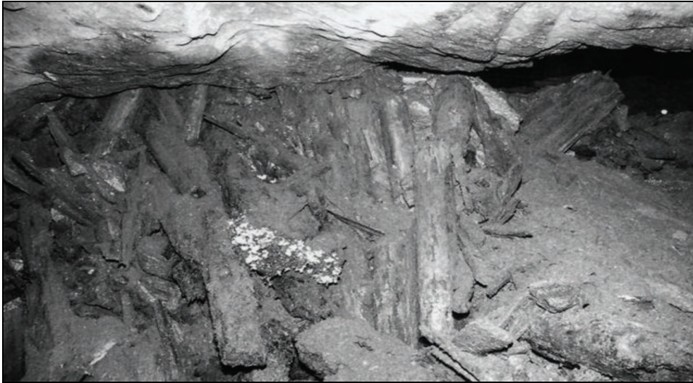
Figure 3. Filling station shaft 302 after opening (view top down).
