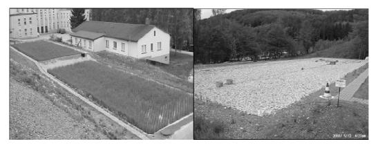
Figure 8: Experimental multi-cell wetland at WISMUT's Schlema mine site (left: plant cells, right: microbiological cell with gravel bed)
