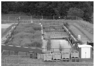
Figure 3: Photograph of the pilot-scale wetland at Poehla
