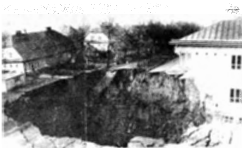
Fig. 7 Photography of a collapse sink
